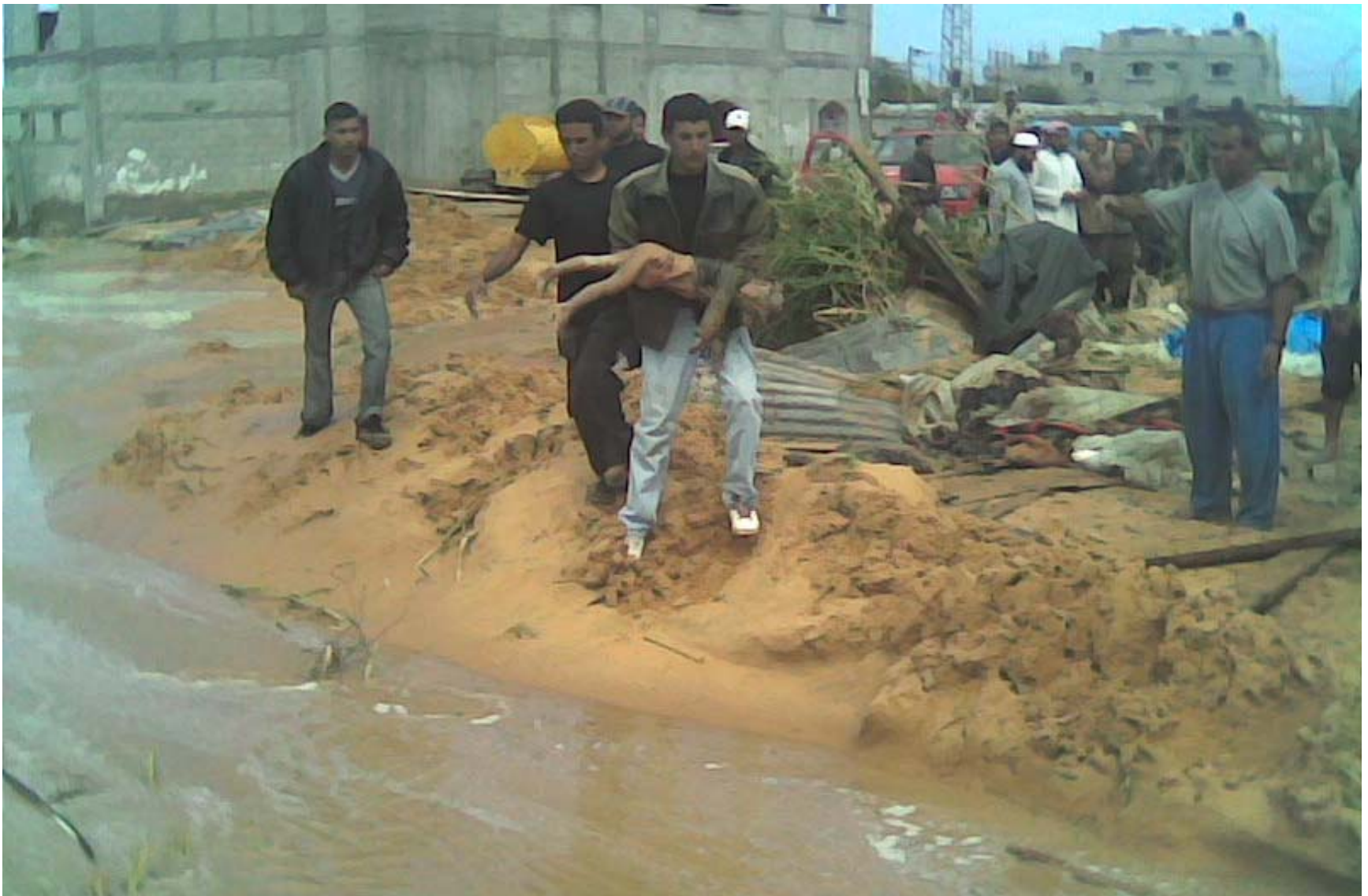
Breach of Sewage Lagoon in Beit Lahia (March, 2007)
